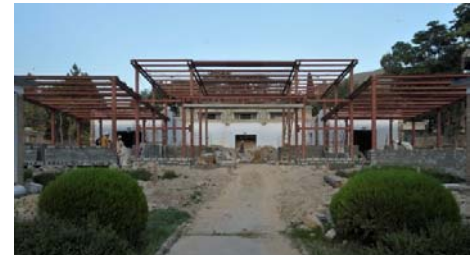
Fig. 9 Block A: steel structure;
